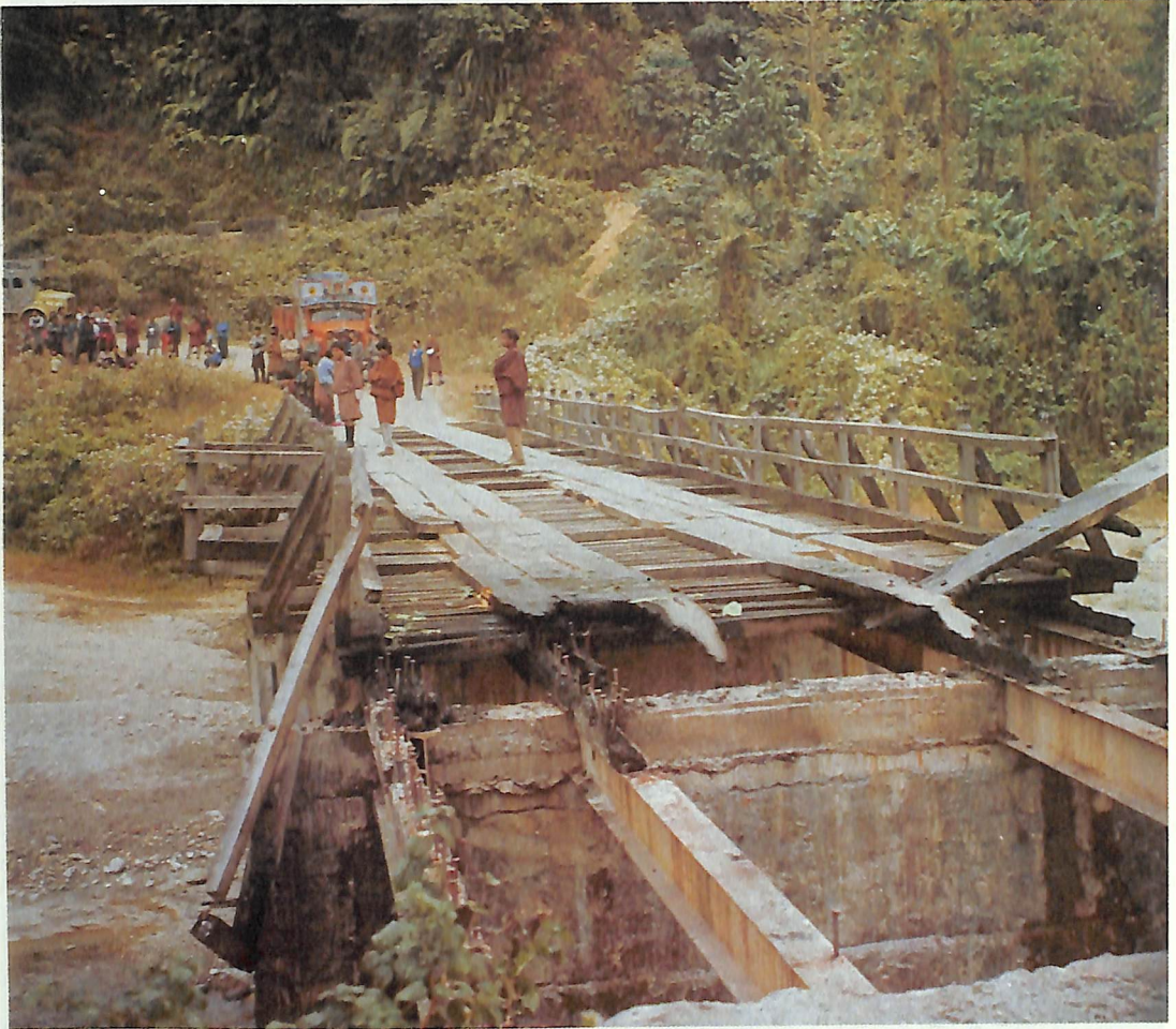
The Kuchi Dyna bridge on the Samchi-Sibsoo highway in Samchi district which was set on fire by terrorists in the early hours of 18 December 1992.
