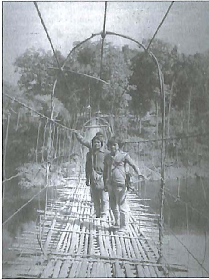
Fig1.6. Cane-suspension bridge (Photo: S.K. Sharma)
