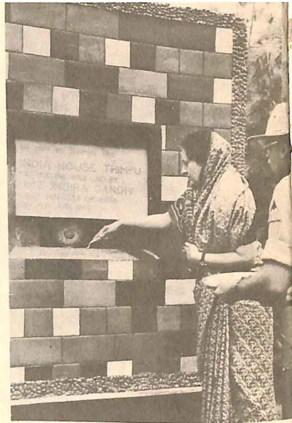
India's Prime Minister Shrimati Indira Gandhi laying the foundation stone of "India House, Thimpu" which will house the office and residence of the India's representative in Bhutan.
