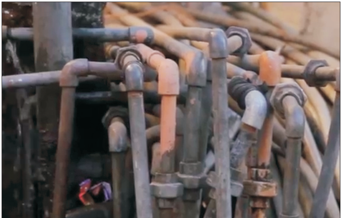
Plate 15: Water Pipe Connection
