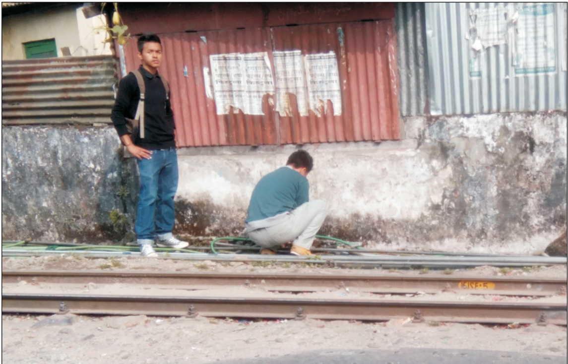
Plate 9: Repairing Pipe Municipal Officials
