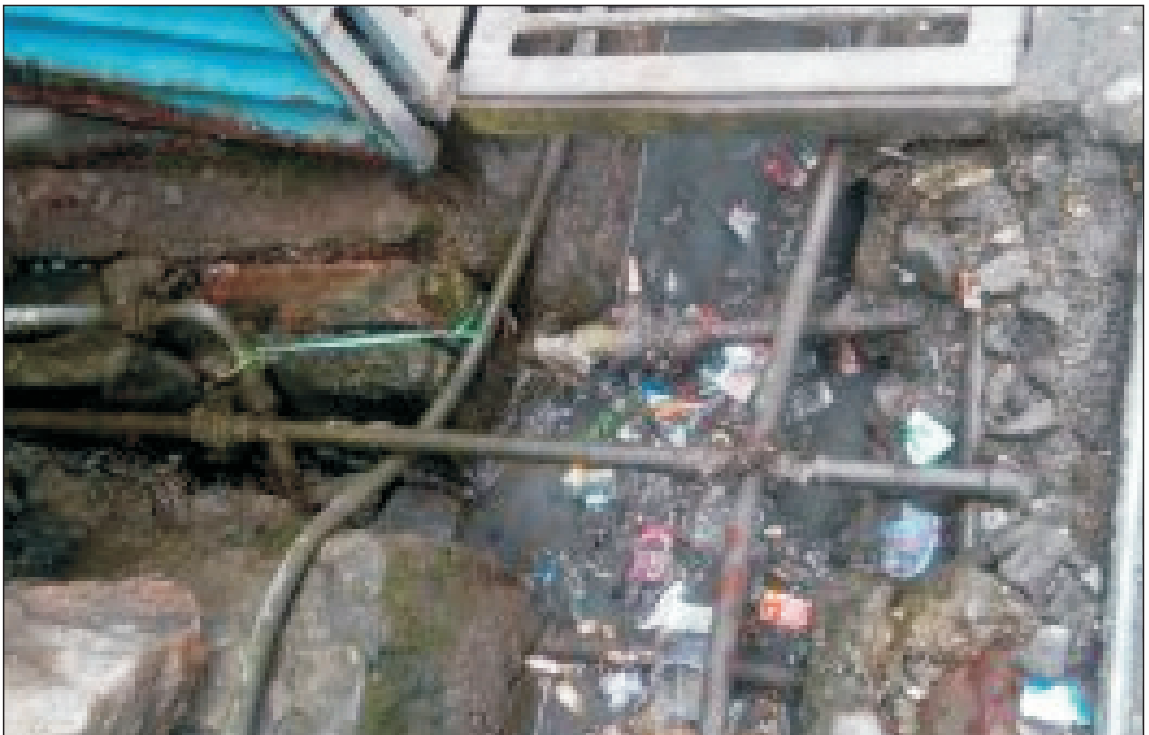
Plate 13: Sewerage Line in Town
