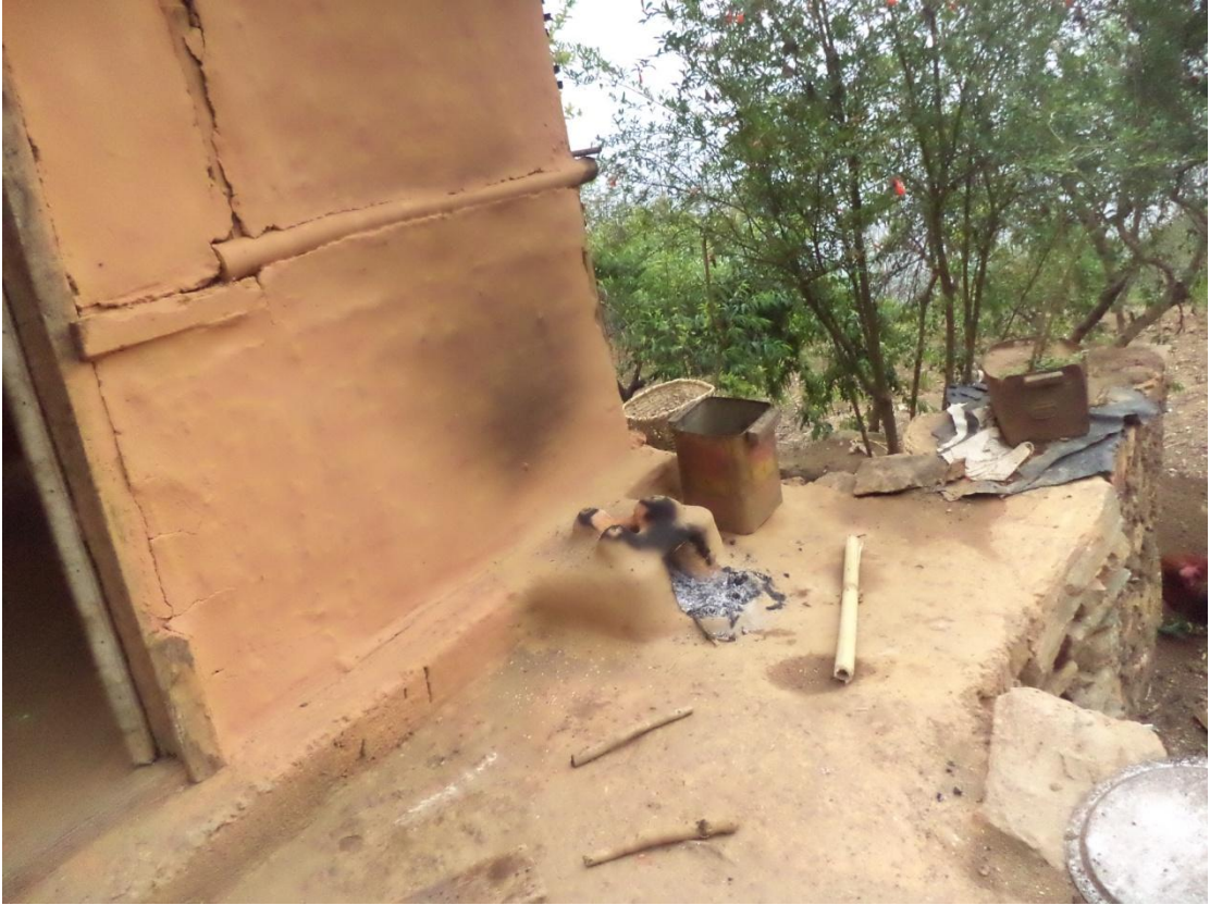
PLATE 2.2: Outside fireplace in Mellidara(Photo- Rashmita Sarkar, April 2017)
