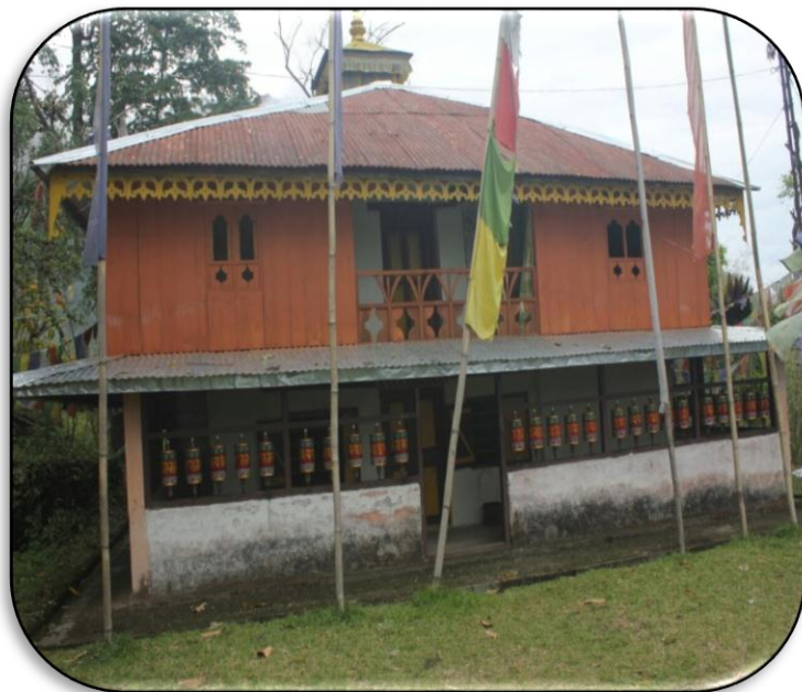
Fig.3.2. Tamang monastery in Malli Dara in South Sikkim established in 1860.
