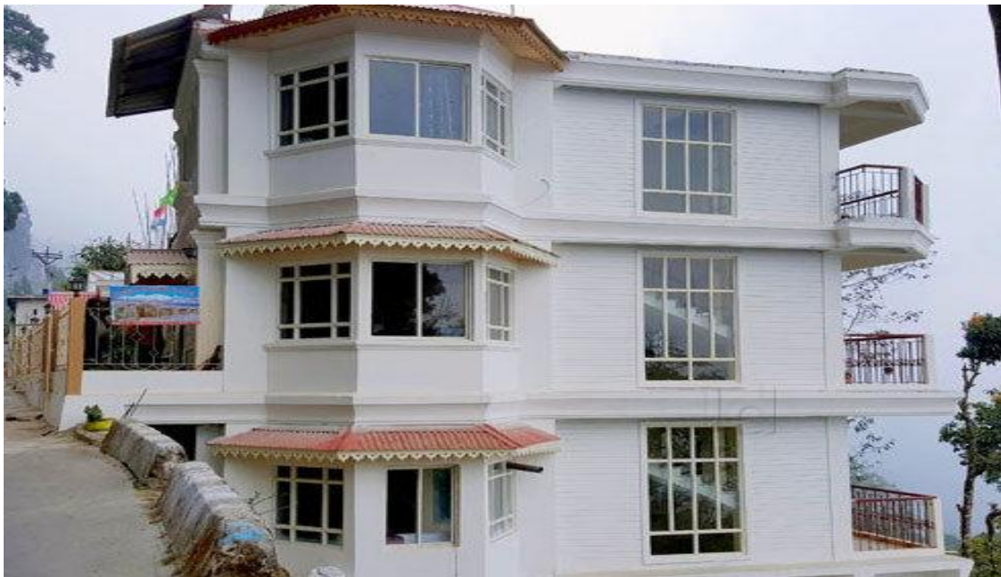
Fig 2.8: Construction of a New Home Stay at Lamahatta
