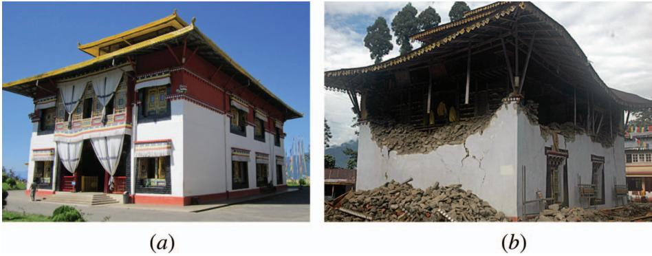
Figure 13. (a) Satisfactory performance of King's monastery in Gangtok (*MSK-VI*) and (b) partial collapse of Ringhem Choling Monastery at Mangan (*MSK-VI*).
