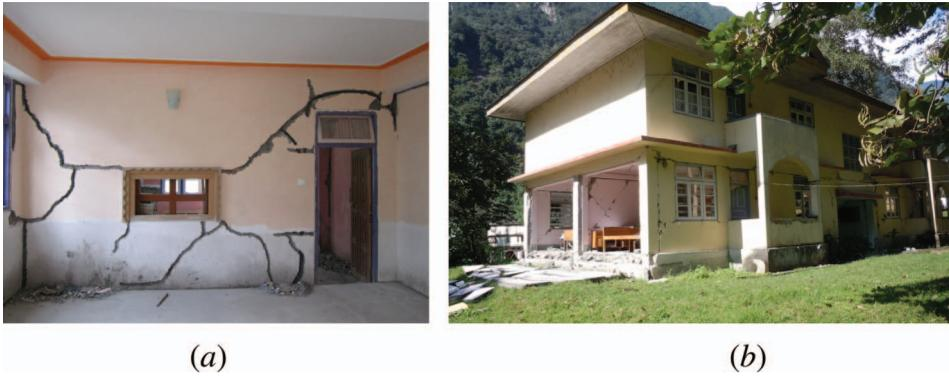
Figure 9. (a) In-plane failure of weak infill masonry and (b) out-of-plane collapse of concrete block masonry walls.
