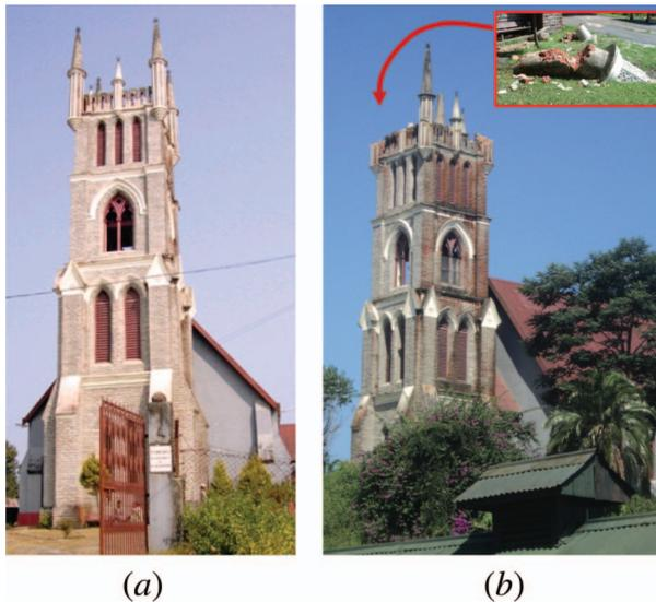
Figure 14. Collapse of brick spires of Mac Farlene Church at Kalimpong (*MSK-VI*): (a) before the earthquake (Photo: <http://mntravelog.com/tag/macfarlane-memorial-church/>) and (b) after the earthquake.
