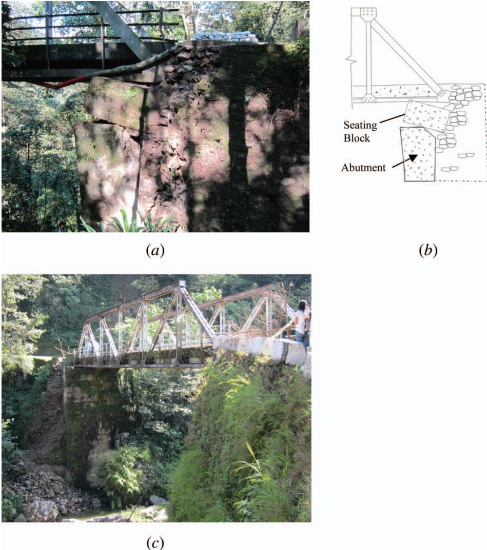
Figure 6. (a) Failure of seating block overhanging the abutment of Plaekhola Bridge, (b) schematic of the failure of seating block at Plaekhola Bridge and (c) damage to the wing wall of steel truss bridge on Raykhola.
