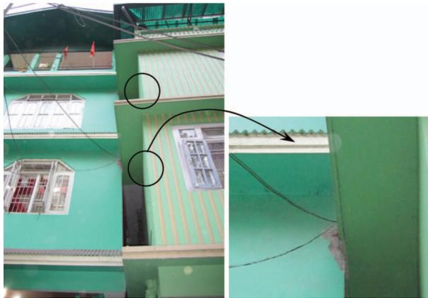
Figure 10. Pounding damage to adjacent buildings at Gangtok (*MSK-VI*).
