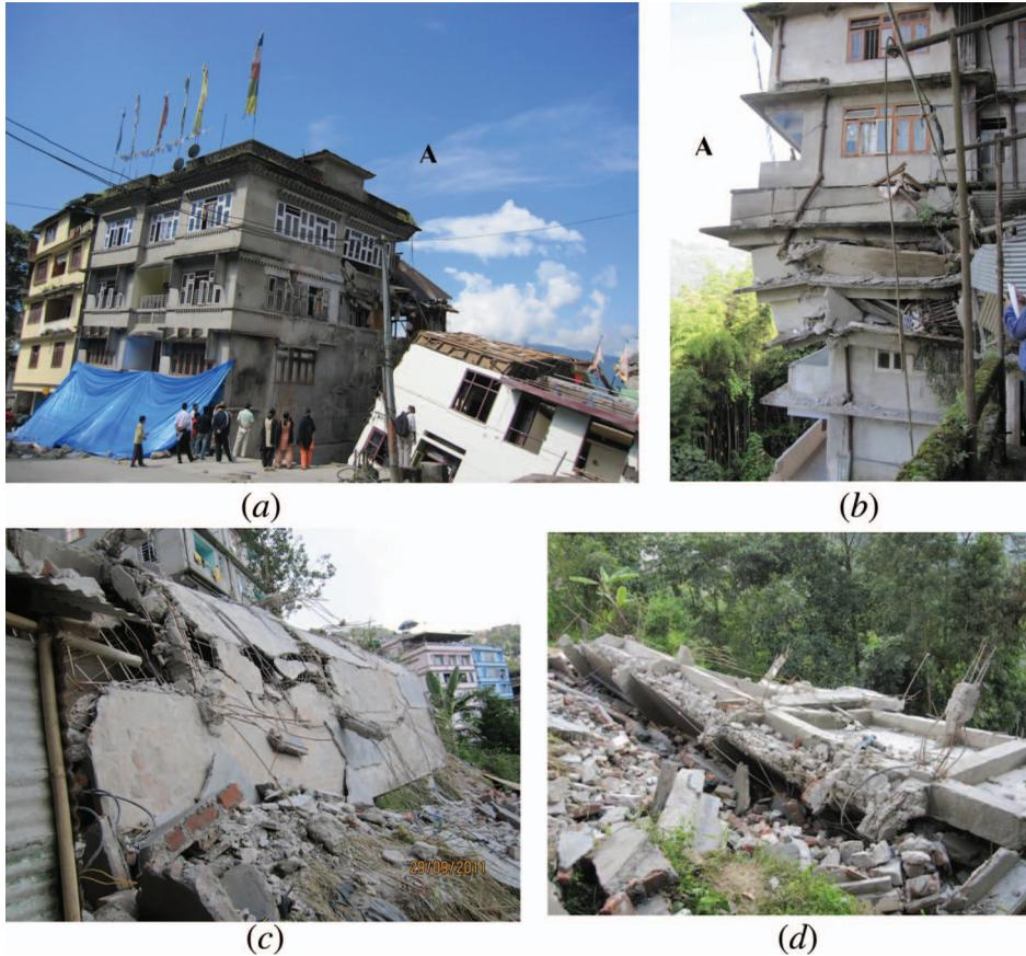
Figure 5. (a) Collapse of two multi-storey buildings at Balwakhani in Gangtok (*MSK-VT*); (b) view of building A, in figure 5a, from backside; (c) and (d) collapse of a five-storey building at Lumshey Basti in Gangtok.
