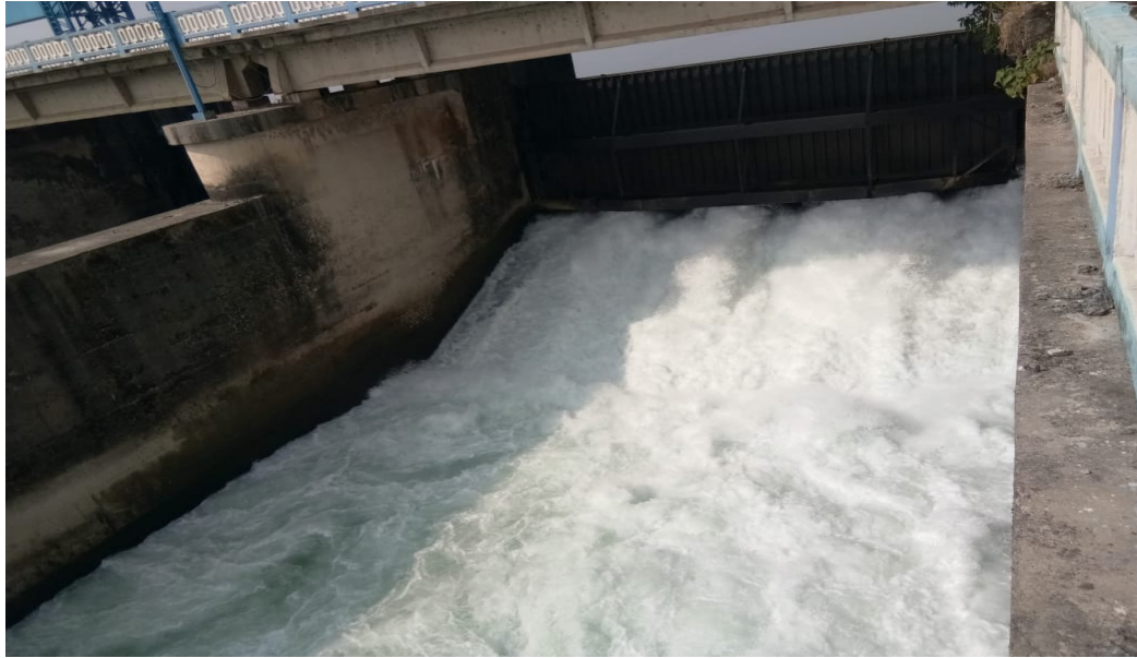
Plate No.1: Canal Fall for Hydropower Generation
