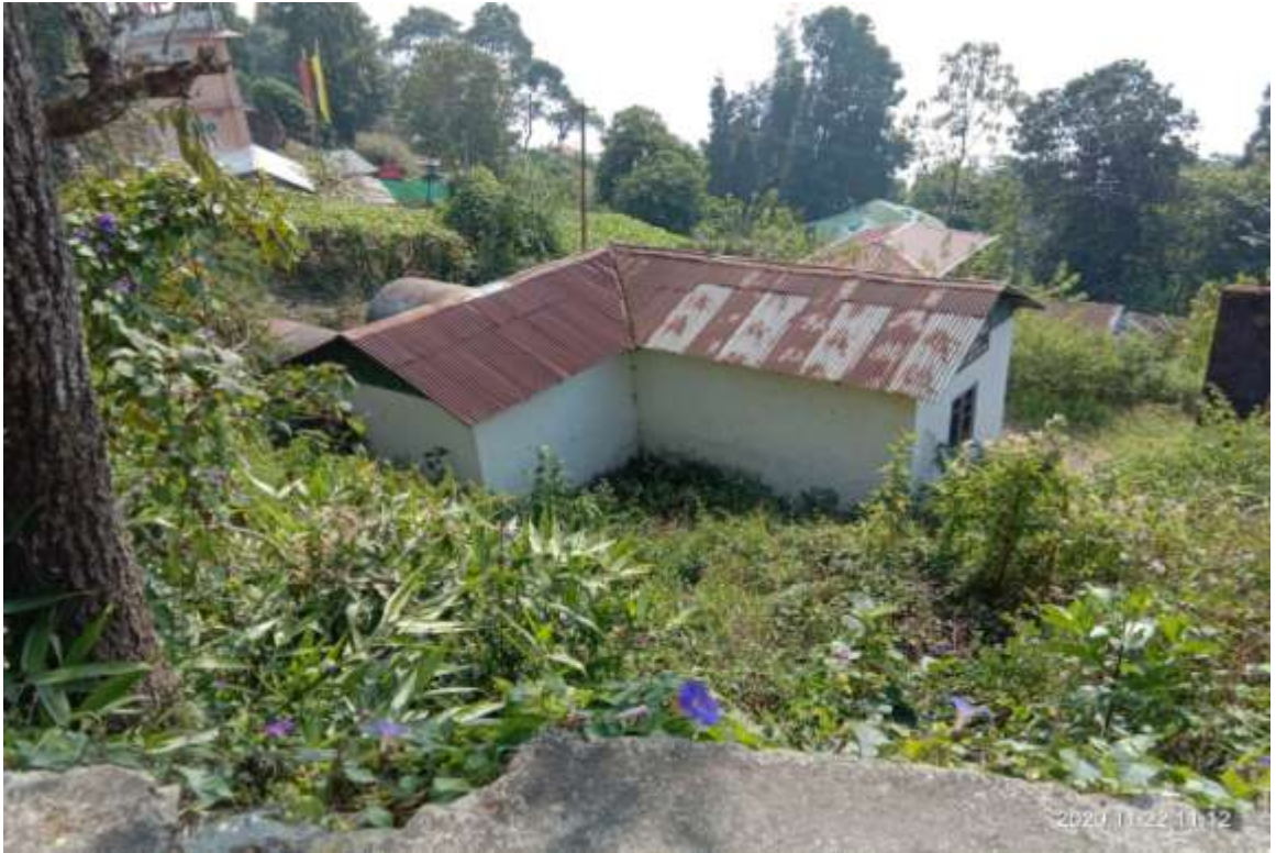
Figure 2.12: Water Filtration Plant of WWD, PHE
