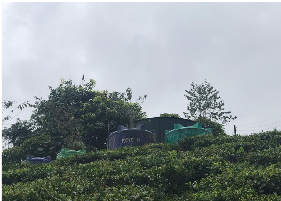
PLATES 11: Setting of water tank in the estate
