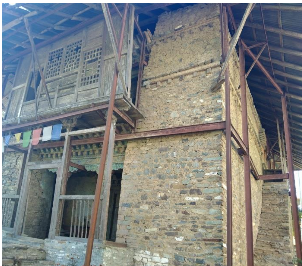
Appendix 13. Pende Wangmu's Palace in Namchi, build in the 17 th century.
